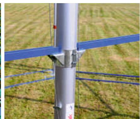
Upper steel powder painted connectors bond cage pillars together
