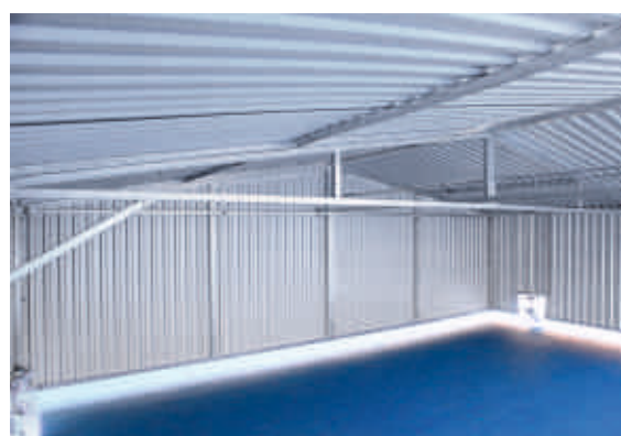
supporting construction made of hot galvanized steel, aluminium-zinc sheet roof and sides
