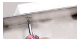
White take-off board, fixed from below, without metal elements on top
