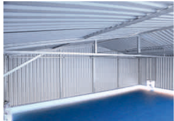
supporting construction made of hot galvanized steel, aluminium sheet roof and sides
